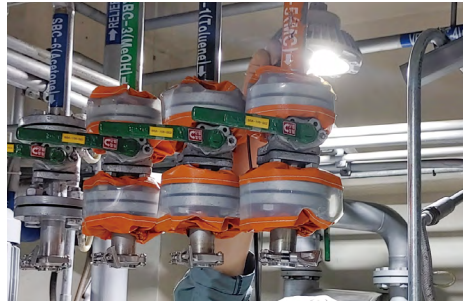
Installation of flange covers on hazardous chemical pipelines
